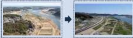
Heightening and strengthening of levees
